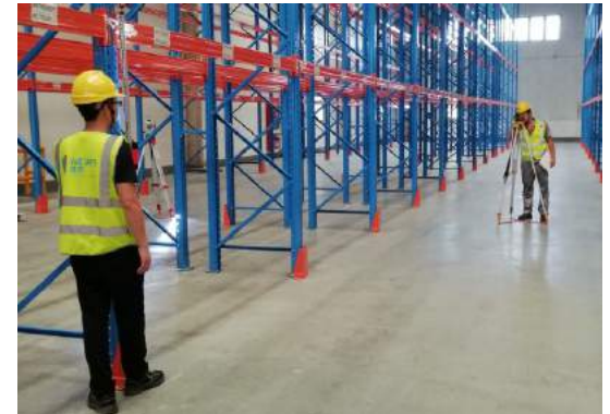
Inspection of Ground Floor Subsidence
