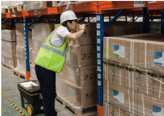
Visual Measurement of Damage to Structural Members
